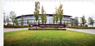
Heifer International Green Building
